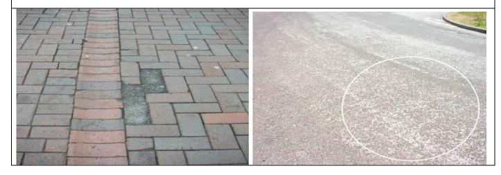
**Condition 3 "Mid-life" =** Signs of defects i.e. cracking, fretting, potholes, subsidence etc – all defects below intervention levels. – **GREEN**
